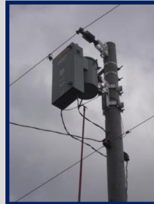
INSTALACION DE TABLEROS ENERGY GUARD JPS - JAMAICA
